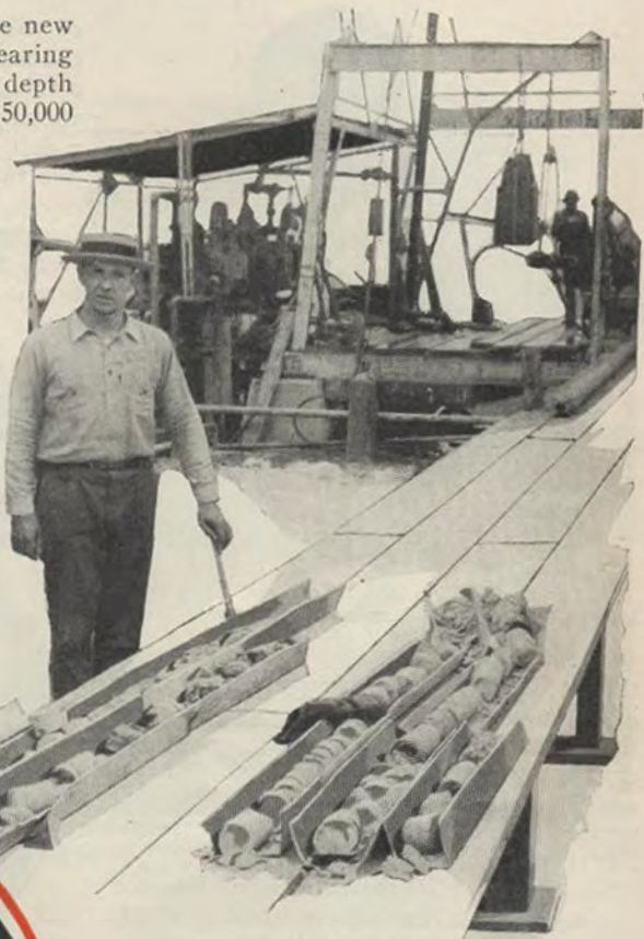
Core Samples from Wells Containing "Bugs"; Pencil Points to a Fault Shown in a Core
